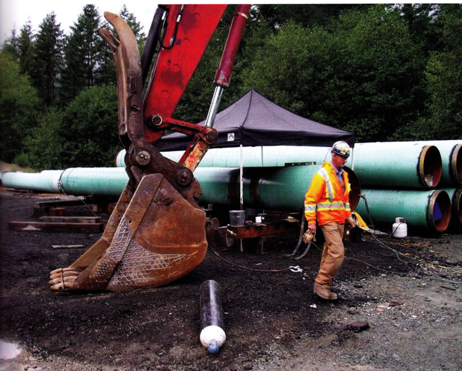
Construction of Canoe Creek Hydro Project Photo by: Tla-o-qui-aht First Nation
